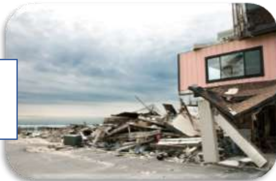
Damage caused by a hurricane.
